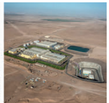
Desalination plant - Agadir
