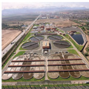
Wastewater treatment plant - Marrakech
